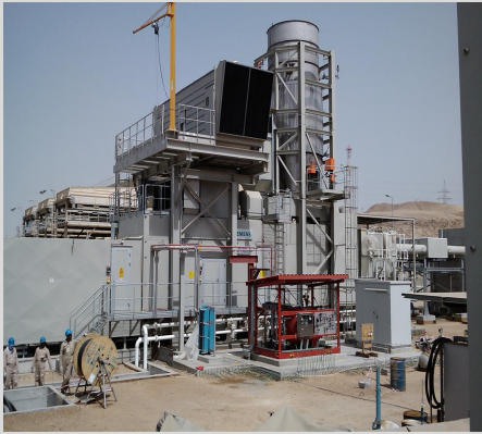
Control, electrical and instrument commissioning of 3 x units of 24MW gas turbines in Saudi Arabia.
